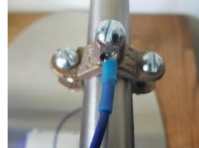
FIG. 4 Rigid Pipe Connection
